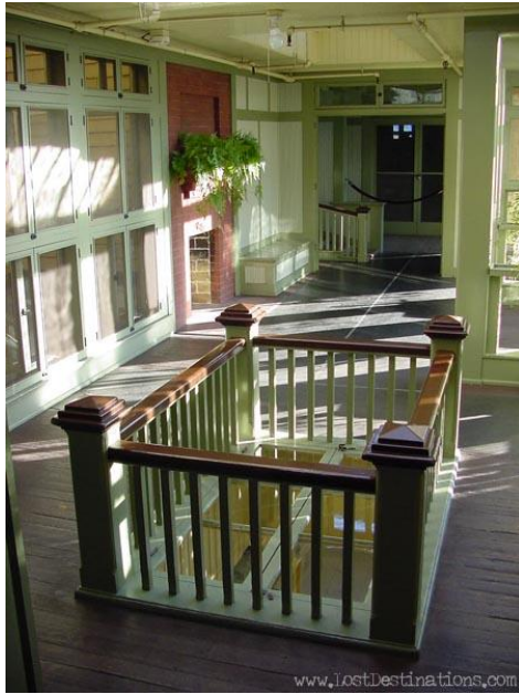
Skylight embedded in the floor
